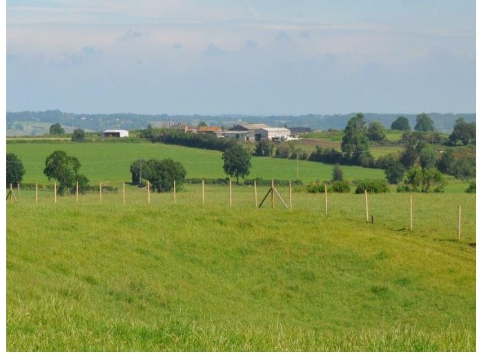
View of the south facing façade and surrounding farmyard, taken from the western edge of field O5.
